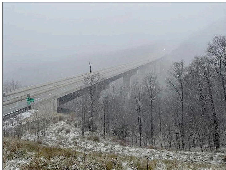
A view of U.S. 48 Corridor H. Photo taken by Paarth Chauhan.
