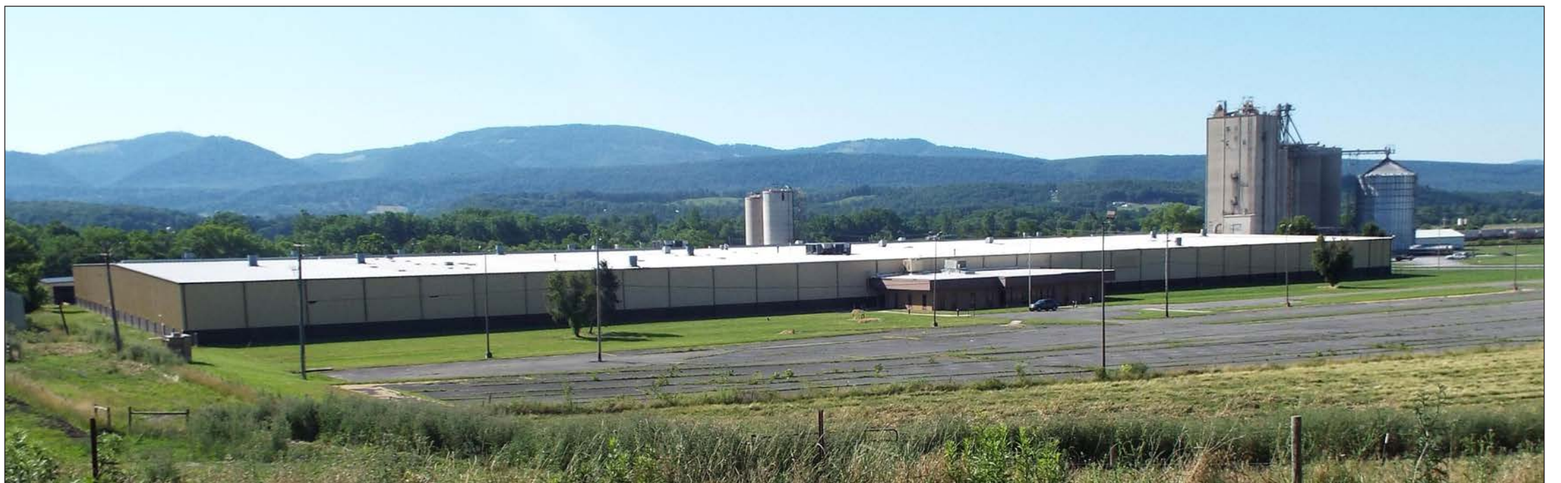
Governor Jim Justice announces German packaging manufacturer Papier-Mettler will locate a new plant in Moorefield. The company acquired the former Allegheny Wood Products building in the Moorefield Industrial Park in May. Although it will start modestly with five positions, at full operation the plant is projected to employ up to 100 people. Idled since Allegheny Wood Products discontinued Hardy County operations, Papier-Mettler acquired this facility in the Moorefield Industrial Park. It will be their first manufacturing operation in the U.S. The company plans to invest $48 million in the project.
